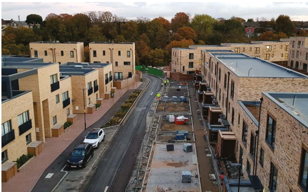
Construction of New Homes
