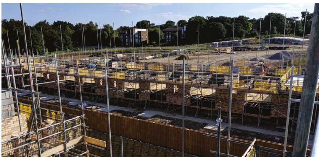
Construction of New Homes (Parcel 10 & 14)
